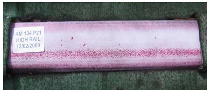
Figure 4 – Dye penetrant for rail surface evaluation
